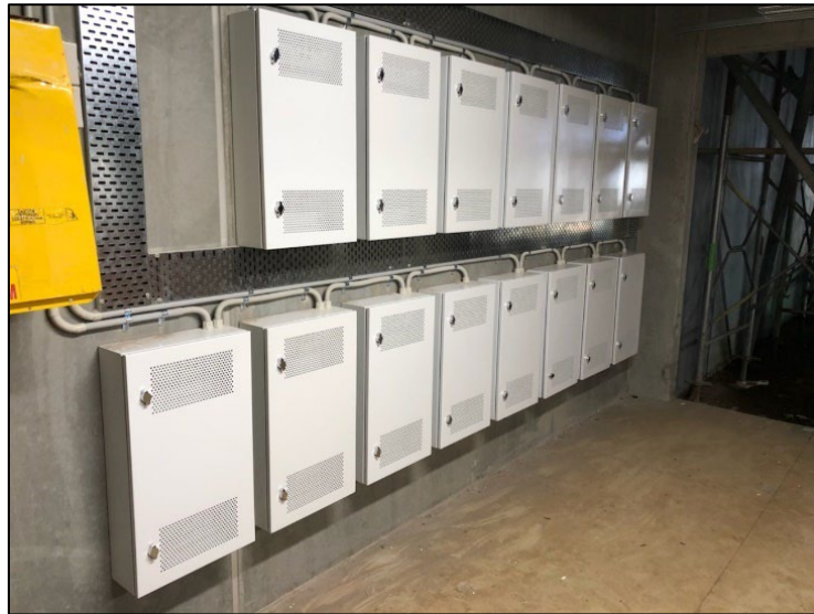
Figure 27. Centrally located NTDs for commercial developments
